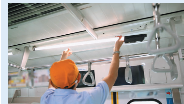
IoTube installation by Tokyu Corporation
