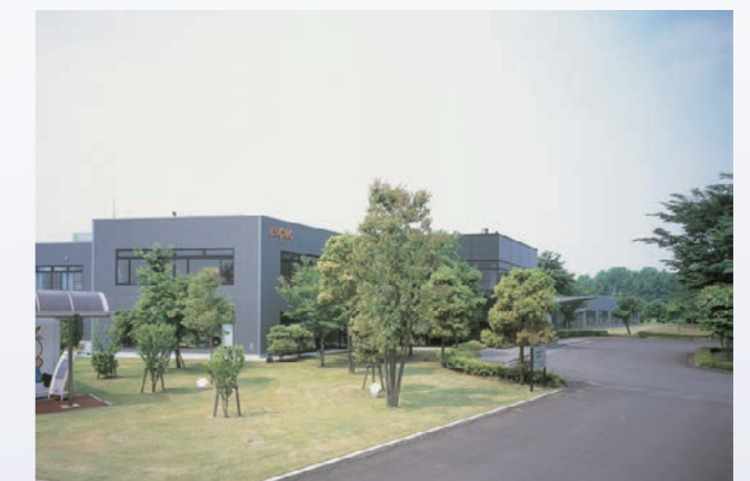
SoftBank Next-generation Battery Lab Image provided by ESPEC Corp.
